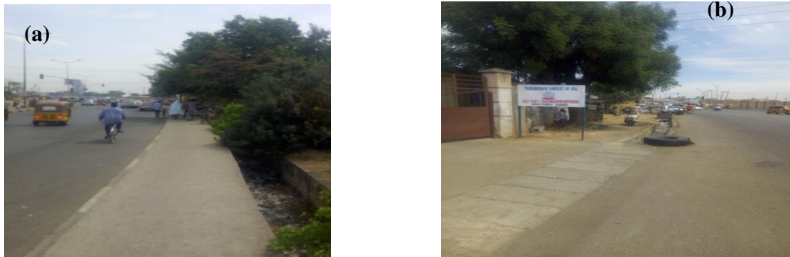
Figure 5. (a) Right hand side of the substation
