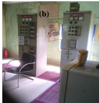
Substation Control Room (b) TR1 and TR2 Control Panels
